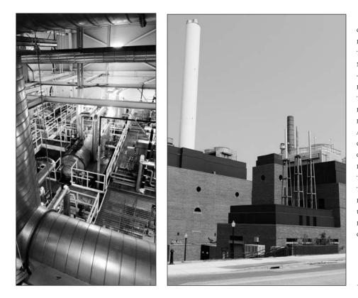
A CUTTING-EDGE CO-GENERATION PLANT OPENED LATE LAST YEAR, ADJACENT TO THE OLD HEATING PLANT. THE NEW PLANT BURNS OIL OR GAS - WHICHEVER IS LESS EXPENSIVE AT THE TIME -- TO TURN TURBINES WHICH CREATE ELECTRICITY. IT IS EXTREMELY ENVIRONMENTALLY SENSITIVE AND COST EFFECTIVE: UNLIKE OLDER SYSTEMS, THE PLANT Converts more than 80PERCENT OF THE HEAT THROWN OFF BY THE HUGE TURBINES INTO A HEAT RECOVERY STEAM GENERATOR. USING THE WASTE PRODUCT TO HELP CREATE HEAT AND CHILLED WATER ON CAMPUS.
