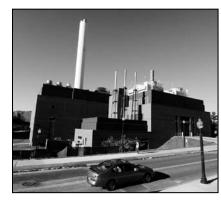
ON THE LEFT, THE CUTTING-EDGE CO-GENERATION PLANT BURNS OIL OR GAS – WHICHEVER IS LESS EXPENSIVE AT THE TIME – TO TURN TURBINES THAT CREATE ELECTRICITY. IT IS EXTREMELY ENVIRONMENTALLY SENSITIVE AND COST EFFECTIVE: UNLIKE OLDER SYSTEMS, THE PLANT CONVERTS MORE THAN 80 PERCENT OF THE HEAT THROWN OFF BY THE HUGE TURBINES INTO A HEAT RECOVERY STEAM GENERATOR, USING THE WASTE PRODUCT TO HELP CREATE HEAT AND CHILLED WATER ON CAMPUS.
